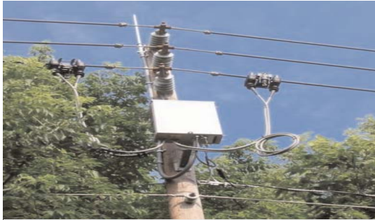
The Griffin 1000 MV delivers speeds of up to 24 Mbps of throughput per MV feeder. This allows backhaul and broadband services to both residential and business customers
